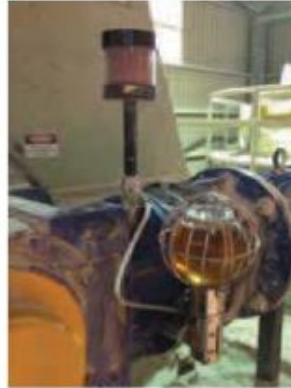
Opto-Matic Closed System Oiler
